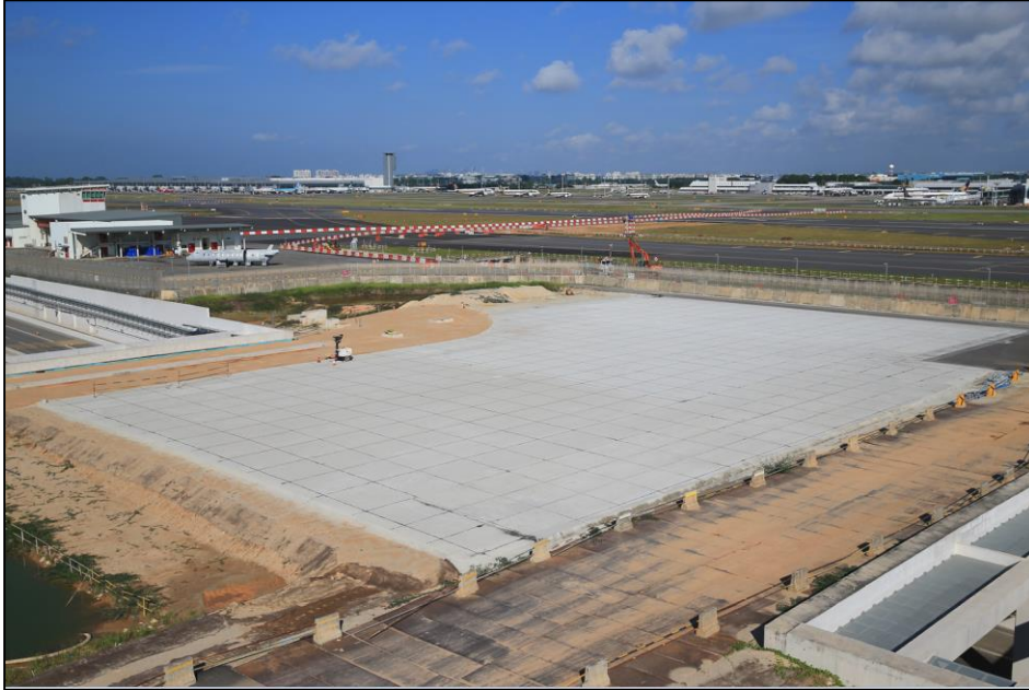
10F CTB with pre-cracking at 3.5m x 3.5m grid
